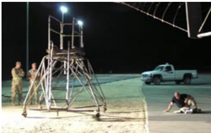
Maintenance personnel assess the damage. The edge of the ramp matting shows the gap area where it started to erode. Notice near the nose of the truck how all the matting was originally next to the ramp, but was dragged to the left.
